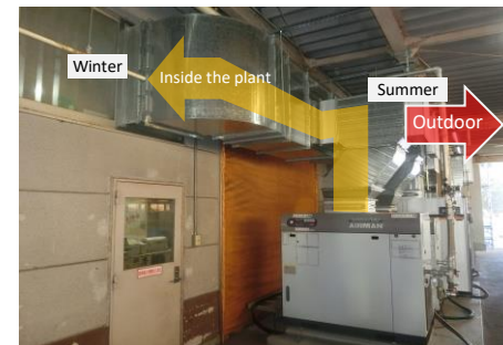
Efficient use of compressor exhaust heat
